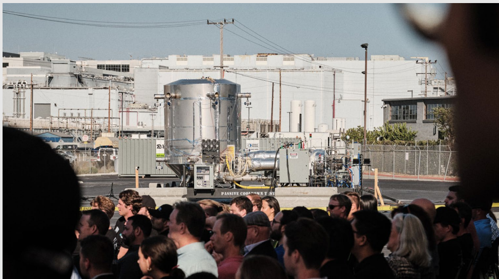
Figure 2 Kaleidos Passive Cooldown Demonstration, 2024 Source: Radiant
